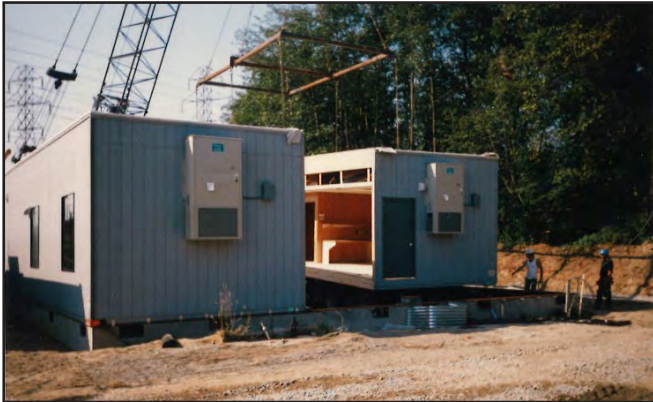
Fig. 10: Installation of trailers used as Brier's City Hall
