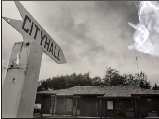
Fig. 17: 1974 City Hall and Substation
