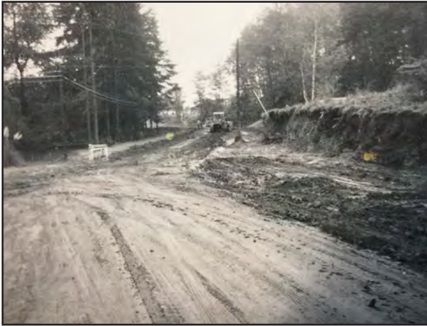
Fig. 15: Sewer extension project
